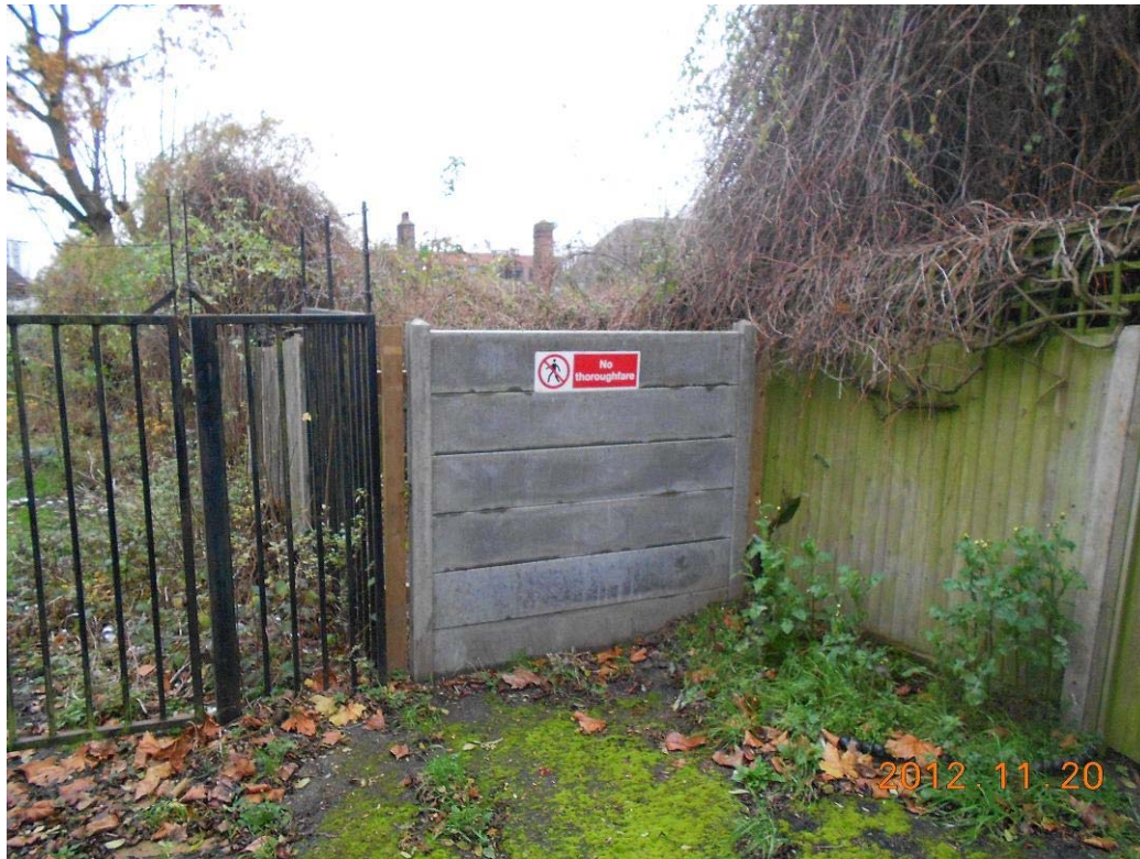
Fence across path at West Heath Road end, beside black painted gate to area around 181 West Heath Road.
